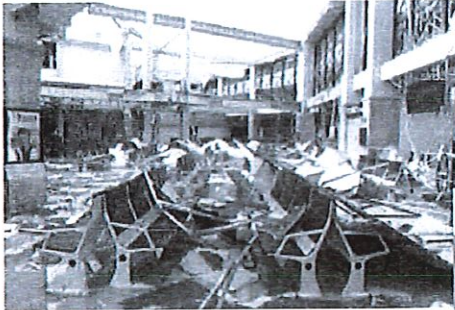
Destruction at Cabo Airport
