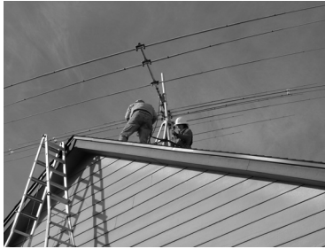
Cheryl, NØWBV helping put up the new beam.
