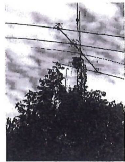
Ria, N2RJ doing antenna work.
