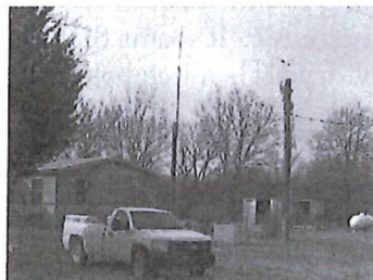
The antenna installation.
