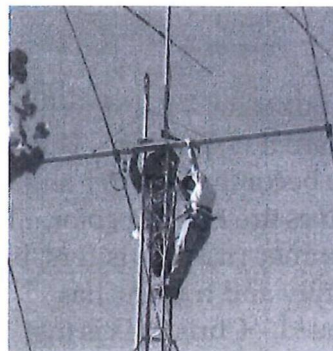
Christine Burke, K0ALT, adds a 17 meter yagi to her 68-ft tower. Neighbor Pat Fitzgerald, KVOK, is helping. Photo by Bob Ludtke, K9MWM.
